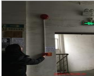
Photo of fire safety equipment Fire alarm testing.JPG
