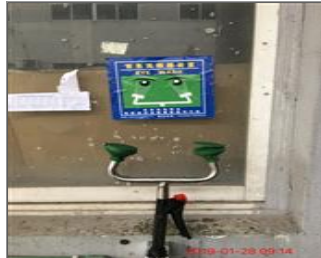
Photo of the inside of the main production hall Eye washing station.JPG
